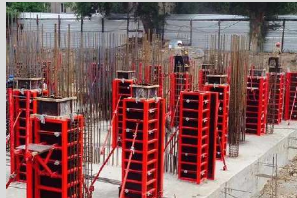
SMALL-PANEL FORMWORK
