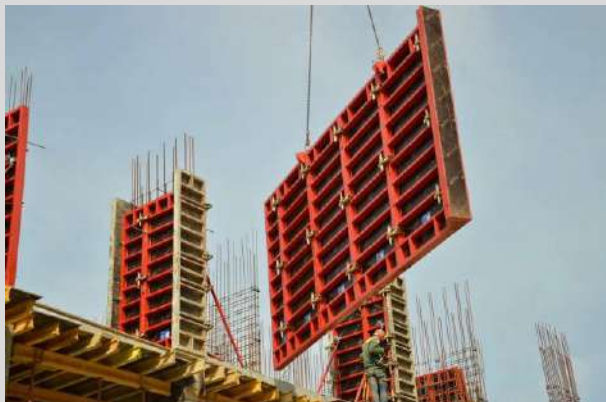
LARGE-PANEL FORMWORK
